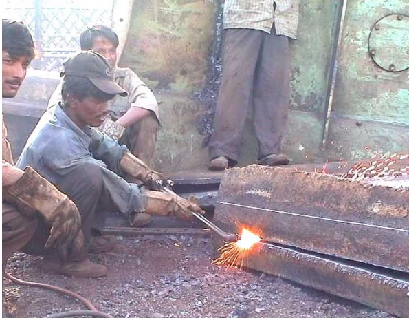
Figure 1. Lacking personal protection equipment
