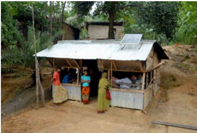
Solar panel on a roof in Bangladesh. Grameen Shakti project.
