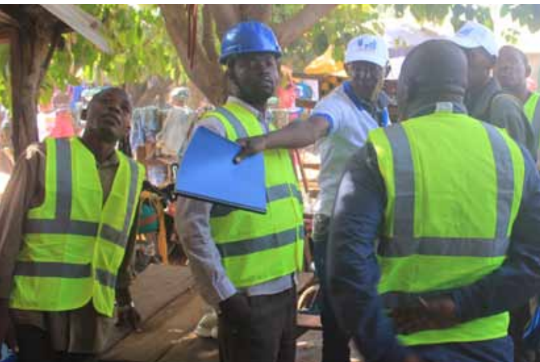
A multi-agency team installs water points, mended latrines and drains in Norassoba, Guinea. PHOTO: ANNE KENNEDY/UNDP
