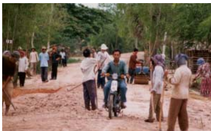
Earthworks by manual labour supported by light compaction equipment, RIIP 2001.
