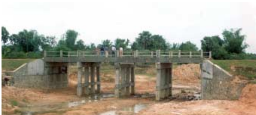
Bridge works by local contractor in Kampot Province, RIIP 2001.
