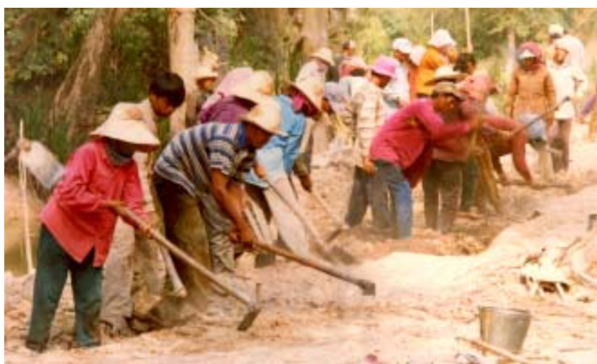
Earthworks by locally recruited labour, Labour-based Rural Infrastructure Works Programme.
