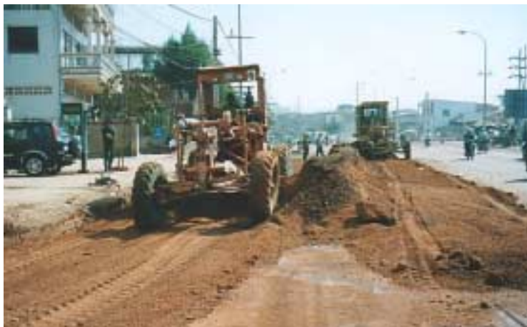
Restoration works on Monivong Boulevard, Phnom Penh 2002.
