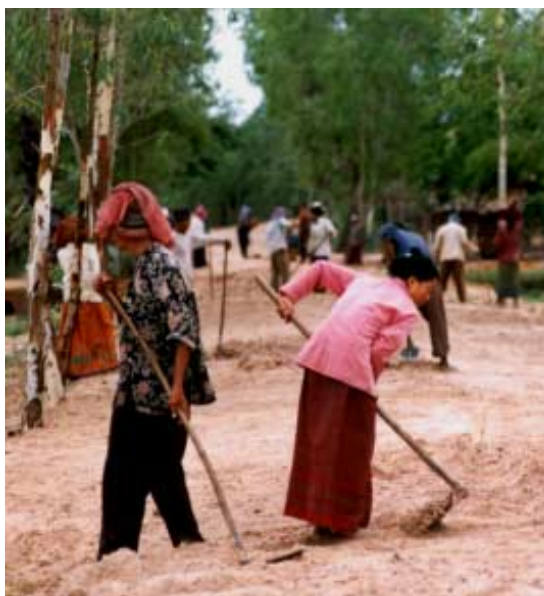
Levelling works by manual labour employed by local contractor, RIIP 2001.
