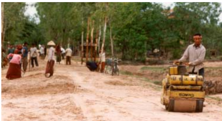
Compaction of earthworks, RIIP 2001.
