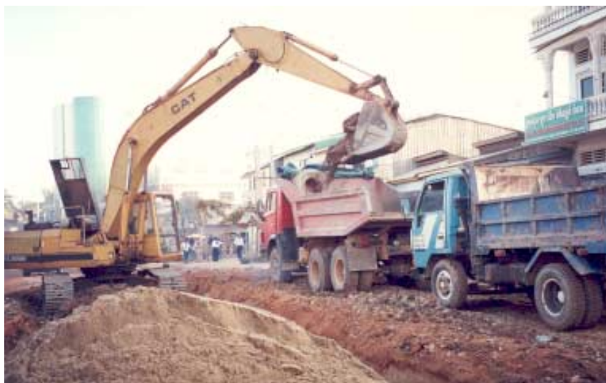
Rehabilitation Works, Monivong Boulevard Urban Road Restoration Project, Phnom Penh 2002.
