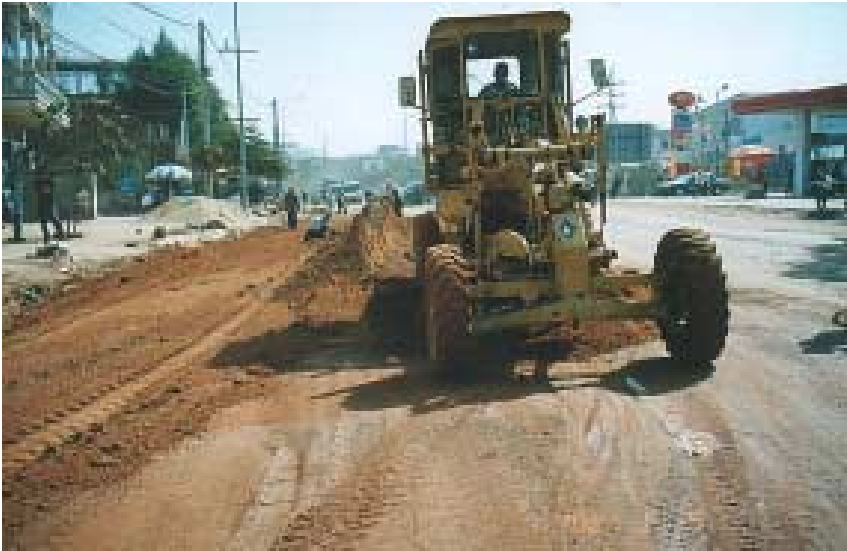
Urban road works, Monivong Boulevard, Phnom Penh 2002.
