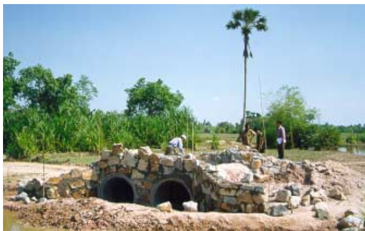
Culvert works by local contractor, Svay Rieng Province, RIIP 1999.
