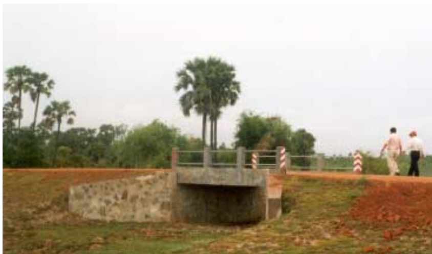
Single Span Bridge constructed by local contractor in Kampot Province, RIIP 2001.
